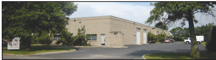
217 Knickerbocker Avenue - Bohemia, NY
