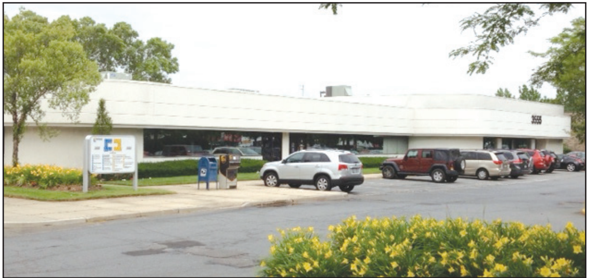
Lakeland Office Condominium, 3555 Veterans Memorial Highway - Ronkonkoma, NY
